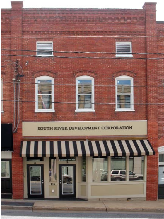
Front of building after renovation. Door to second floor on left. Living room space is at the front of the building.
